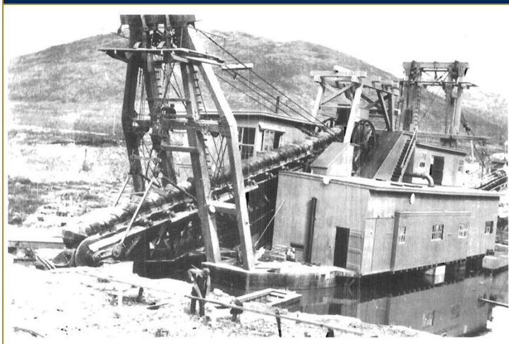
Photo Description: The Yukon Gold Company's 170-liter (6 ft 3 ) capacity Yuba dredge in its construction pit on upper Flat Creek, August 1912. This dredge efficiently mined rich pay for seven seasons and was the Iditarod-Flat District's most successful mining venture. (Bundtzen, 1992)
