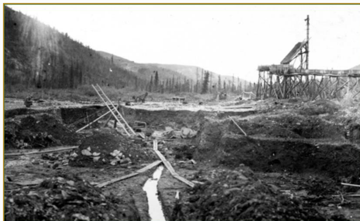
Photo Description: Historic placer mining operation on Flat Creek in 1913. Miners are removing shallow overburden by hand to expose gold-bearing gravel near bedrock.
