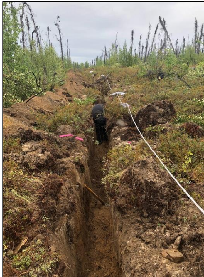
Figure 36. Trenching at Area 7.
